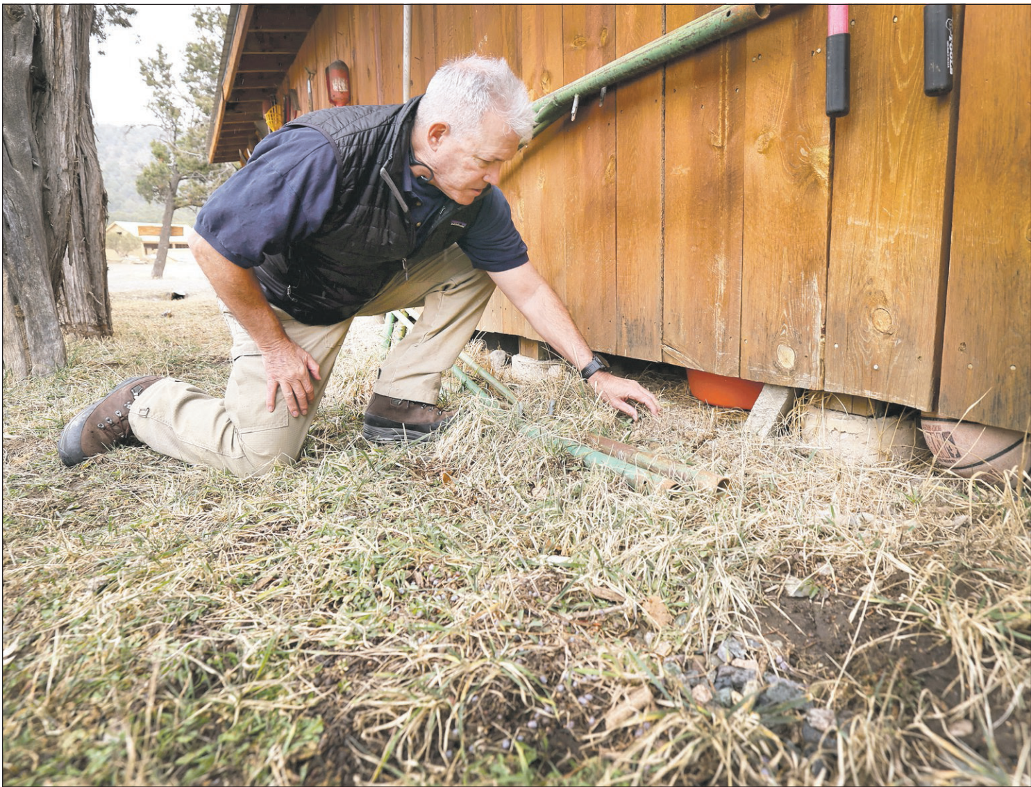
Paul Valdez, Upper Pine River Fire Protection District's wildfire coordinator, shows how fire embers can get under the siding of a building and start a fire. Covering gaps like these with one-eighth inch or smaller wire screens can prevent embers from infiltrating a home.
