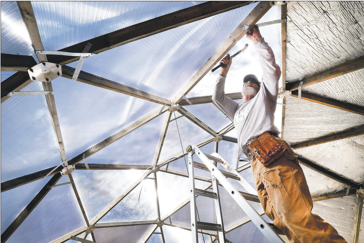
ABOVE: Jim McCarroll volunteers his time helping to build a grow dome on Sept. 24 in Vallecito. TOP: Joey Martinez, with Willis Contractor, works on the dome.
