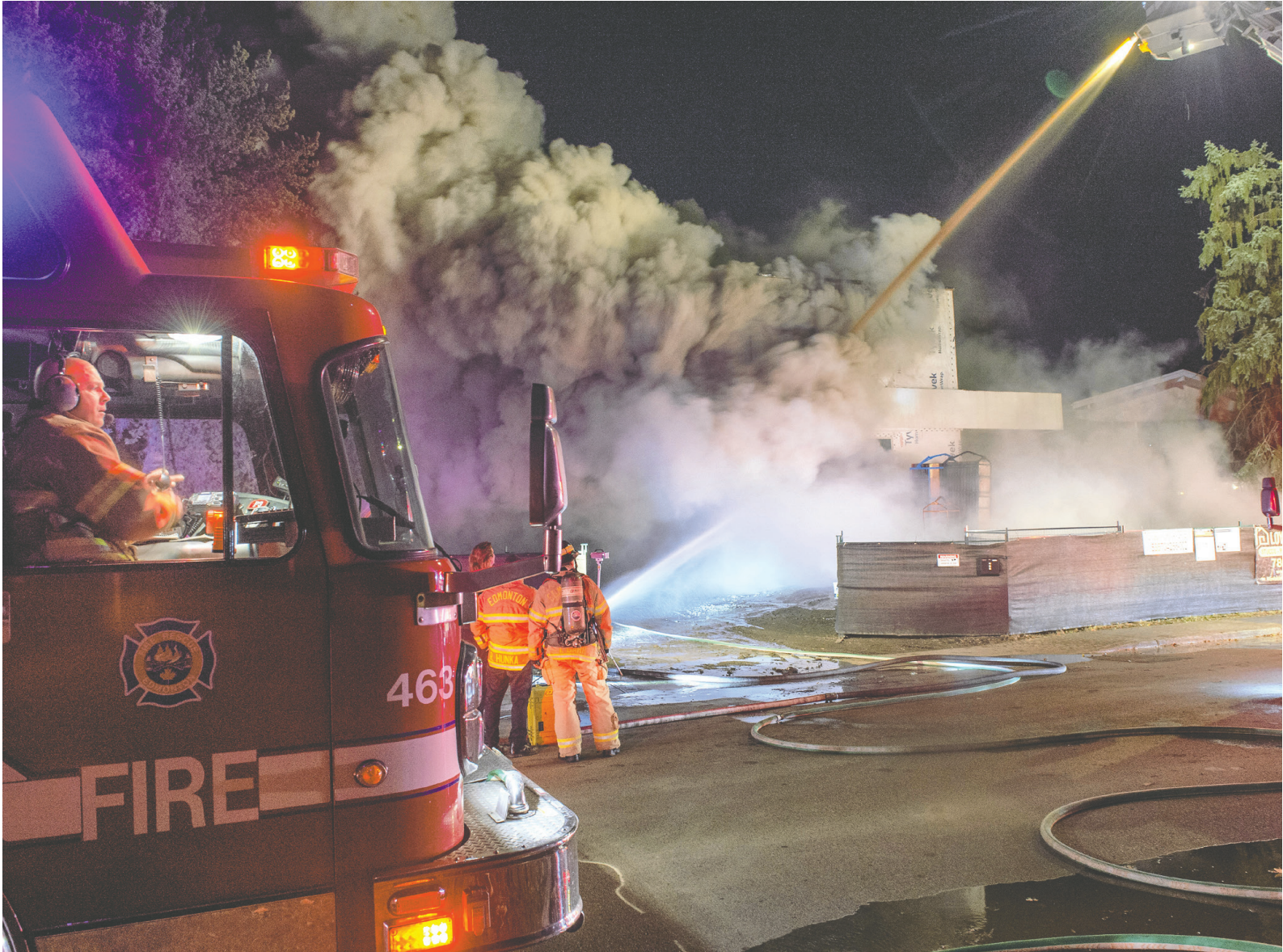
Thick smoke billows from what remains of a single-family infill home under construction on Saskatchewan Drive early Monday morning. The fire is the sixth to hit infill projects in the city in the last few weeks. Four have already been declared arson. SHAUGHN BUTTS
