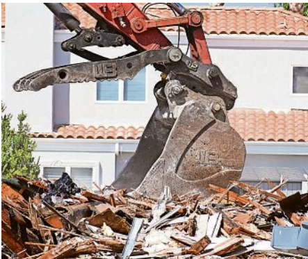
Workers at Oxnard’s Fisherman’s Wharf demolish structures on Sept. 14 in a project designed to lead to the opening of a Karls Village in 2028.
