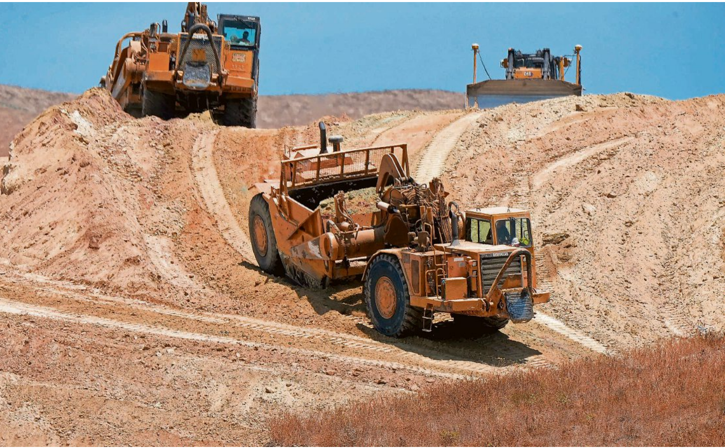
Site grading is currently underway at the former Lost Canyons Golf Club in Simi Valley July 24. The course has been closed for the past 10 years and is being redeveloped with more than 300 new homes. JUAN CARLO/THE STAR
