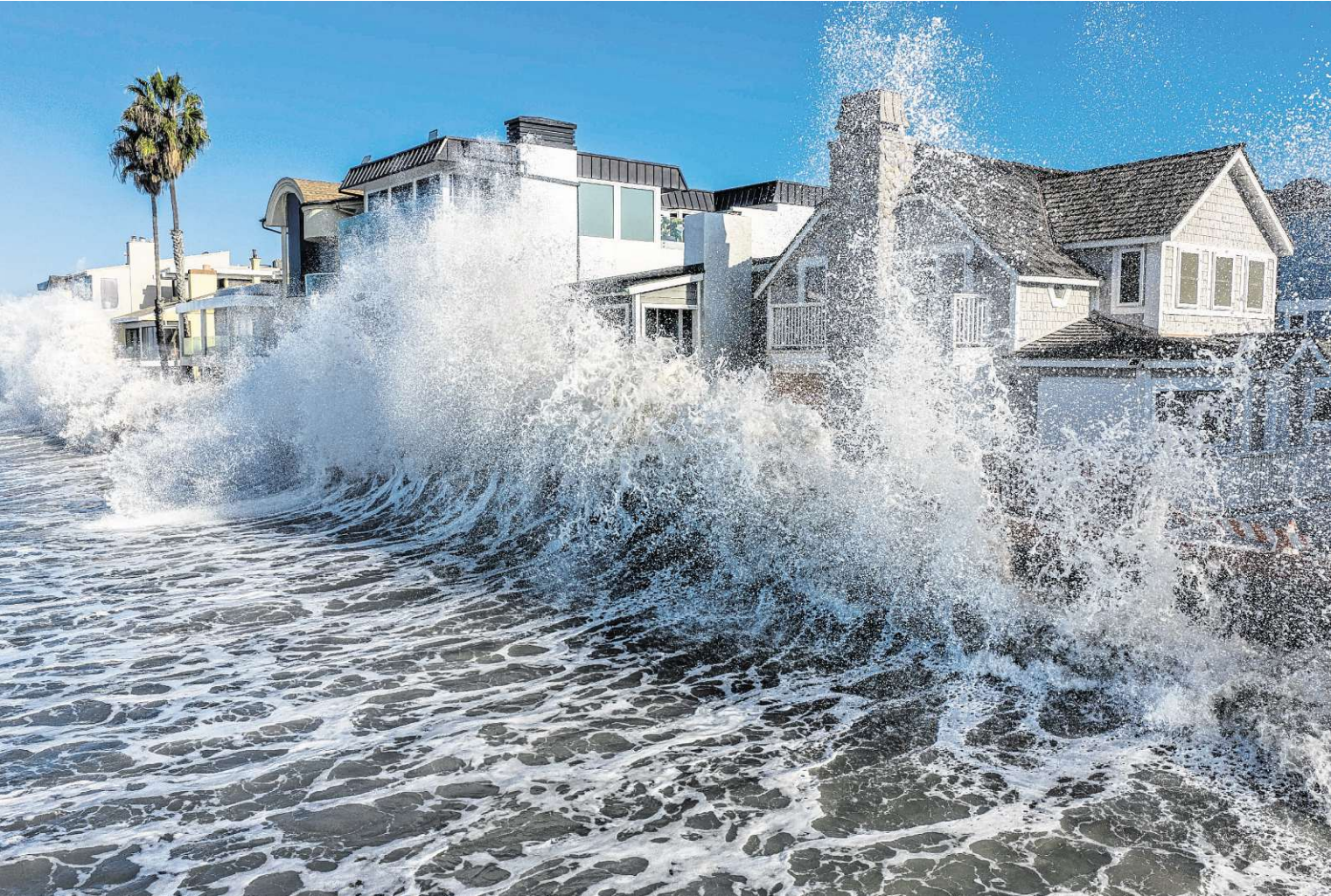
Allen J. Schaben / Los Angeles Times A powerful wave crashed against seawall boards and damaged beachfront homes along the Long Beach Peninsula on Thursday ahead of Tropical Storm Rachel's arrival.
