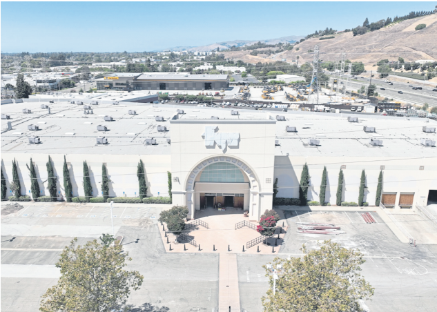
Fry’s Electronics shut down in 2021, leaving large spaces like this one in Fremont vacant. It is being marketed toward AI or industrial reuse. JANE TYSKA — STAFF PHOTOGRAPHER
