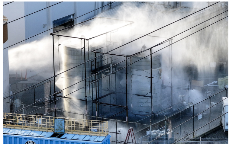
A pressurized tank filled with methyl methacrylate is sprayed with water at GKN Aerospace in Garden Grove on Saturday. Crews have confirmed a crack in the tank. JEFF GRITCHEN — STAFF PHOTOGRAPHER
