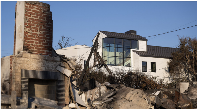
A house behind the chimney of a destroyed Pacific Palisades home had a metal roof without eaves, helping it to withstand January's fire. Drew A. KELLEY STAFF PHOTOGRAPHER
