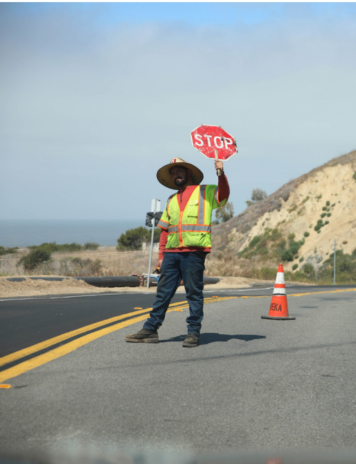
A worker temporarily halts traffic for roadway repairs along a portion of Rancho Palos Verdes Drive South vulnerable to landslides.
