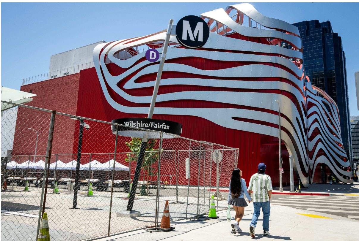
People pass the entrance to the underground L.A. Metro D Line's Wilshire/Fairfax station on Thursday just before the Petersen Automotive Museum on Wilshire Boulevard. PHOTOS BY SARAH REINGEWIRTZ — STAFF PHOTOGRAPHER
