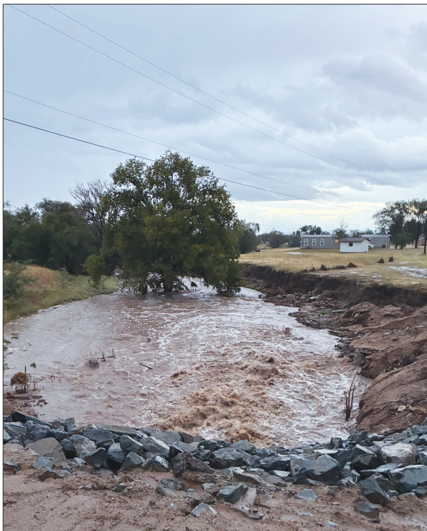
Stormwater flows through a drainage channel following a recent downpour that caused localized flooding in Chino Valley in October 2026. (Town of Chino Valley/Courtesy)
