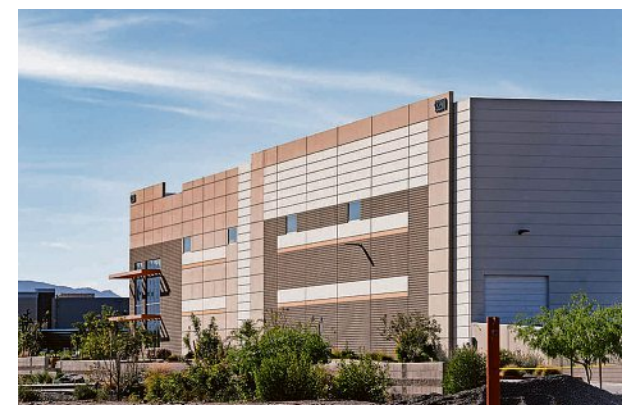
The Department of Homeland Security bought a warehouse near Dysart Road and Sweetwater Avenue in Surprise for more than $70 million in January. However, the idea of an ICE immigration center near neighborhoods and schools has drawn backlash. DIANNIE CHAVEZ/THE REPUBLIC FILE
