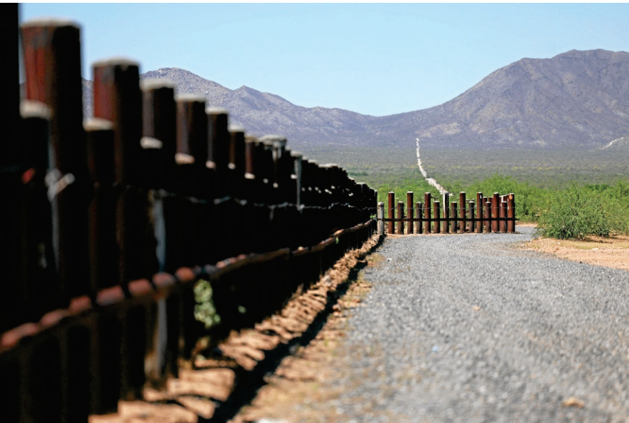
According to the government, the contract for miles of new border fencing in Arizona was awarded last month, with design work starting this month. Construction activities are not anticipated to start before Oct. 12.
